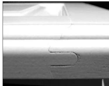
Example of end joint separation
