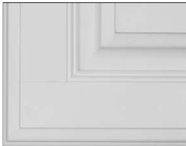
Example of front joint separation
