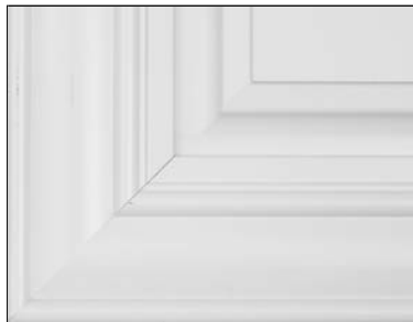
Example of front joint separation
