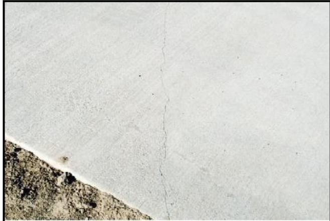
The photo above is an example of a hairline crack, which is not covered, unless the opening is wider than 1/4"
